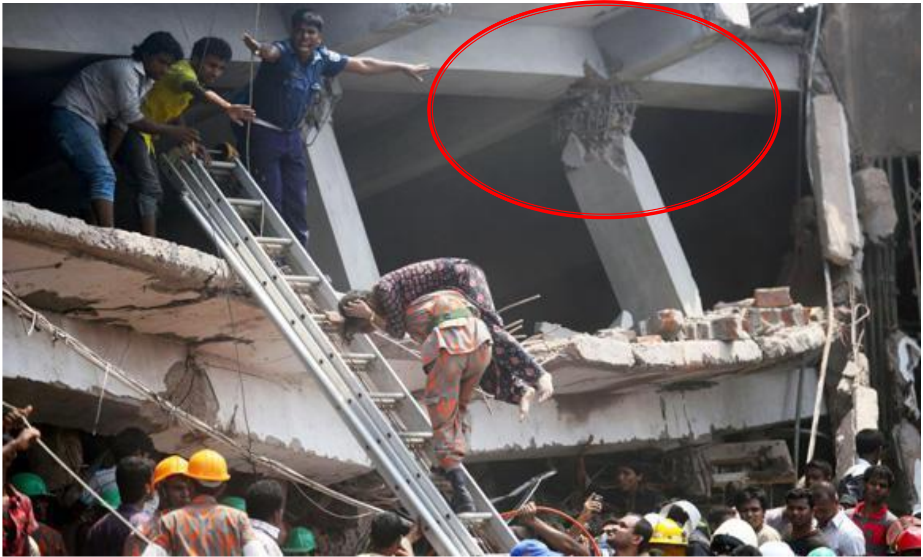
Bulging out concrete near column and beam joints
