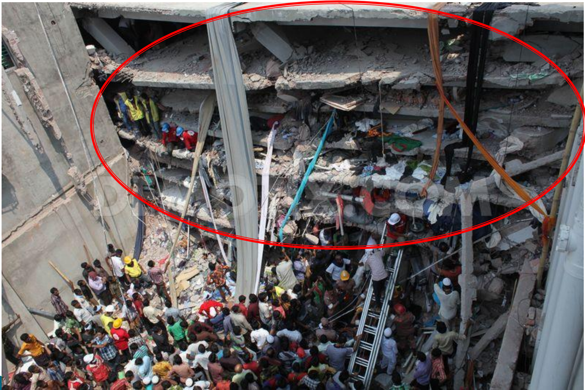
Columns of all floors collapse
