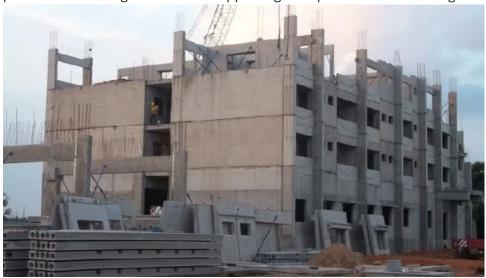
requirement of modular rooms in superstructure makes the precast concrete technology effective due to repetitions and volume.
